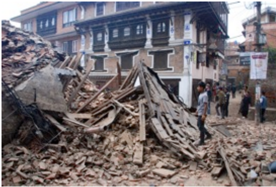
Damage in Swatha Square in Kathmandu. Photo courtesy of Edyta Stepczak
