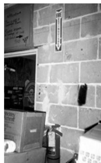
Blocked extinguisher
